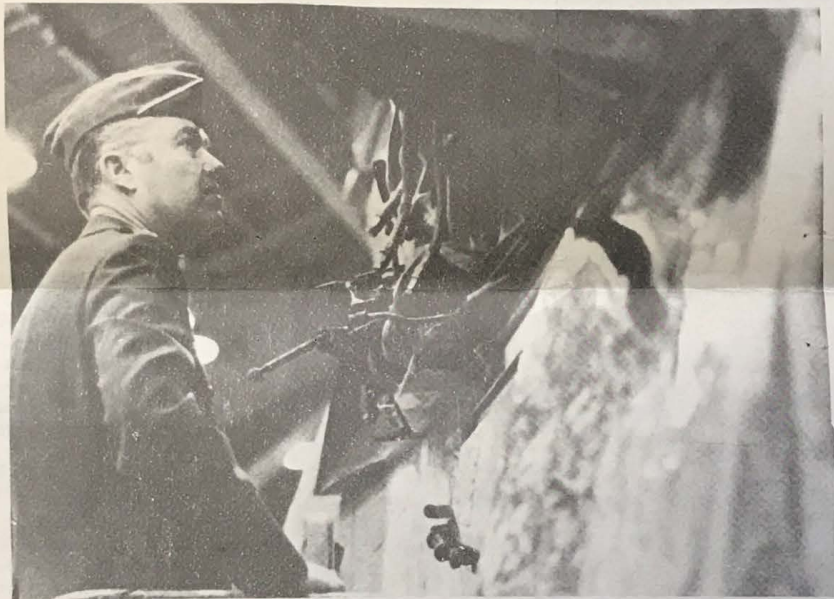
ALC COMMANDER, Maj. Gen. Carl G. Schneider visits the 507th and examines the wing attach points of an F-105 during a wing's-off inspection.
